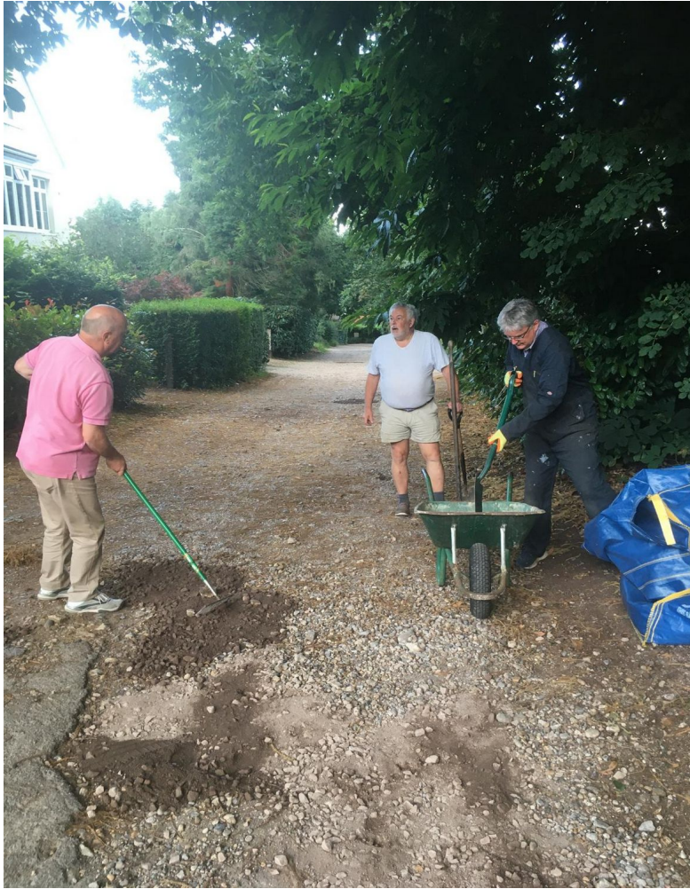
Application of Type 1 filling to potholes
