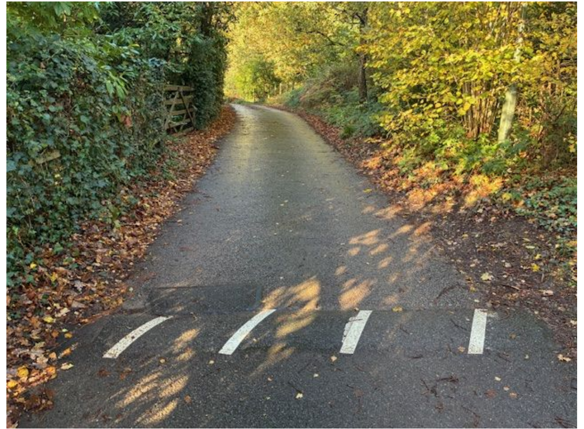
White hatched lines added to all speed bumps
